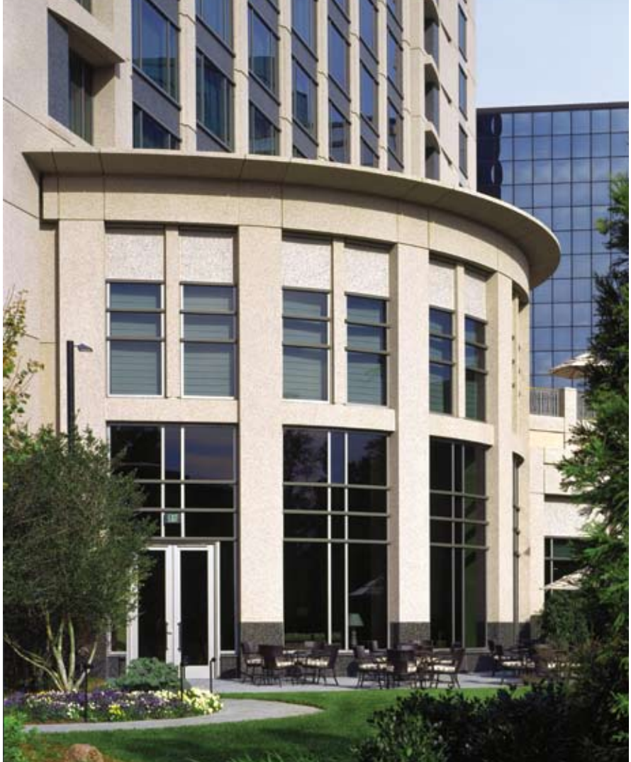
Architectural precast concrete panels were used to clad the InterContinental Hotel in Atlanta because they could replicate the look of stone economically and could be erected quickly, saving time and money.
