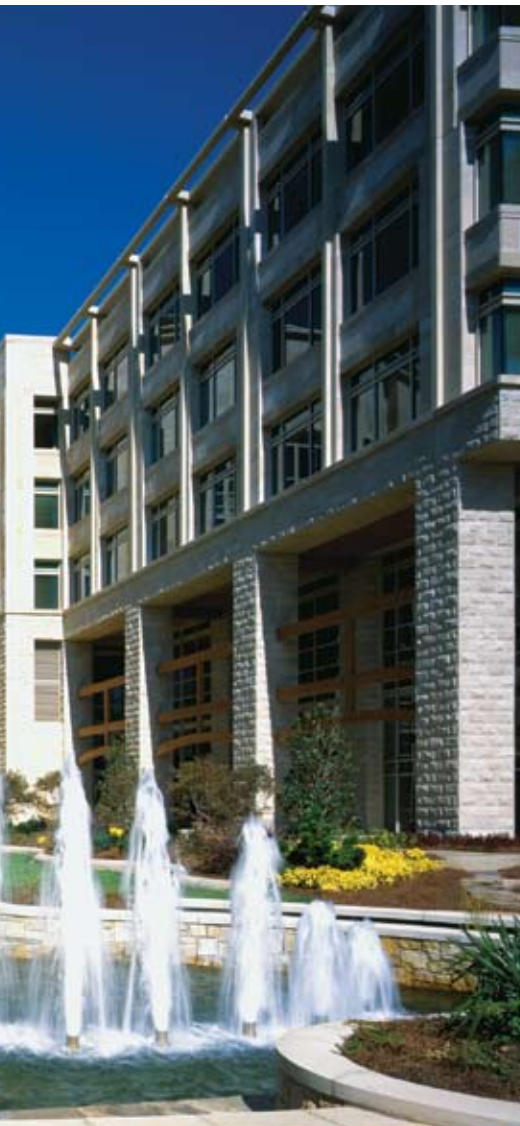
Architectural precast concrete panels were used to clad the InterContinental Hotel in Atlanta because they could replicate the look of stone economically and could be erected quickly, saving time and money.
